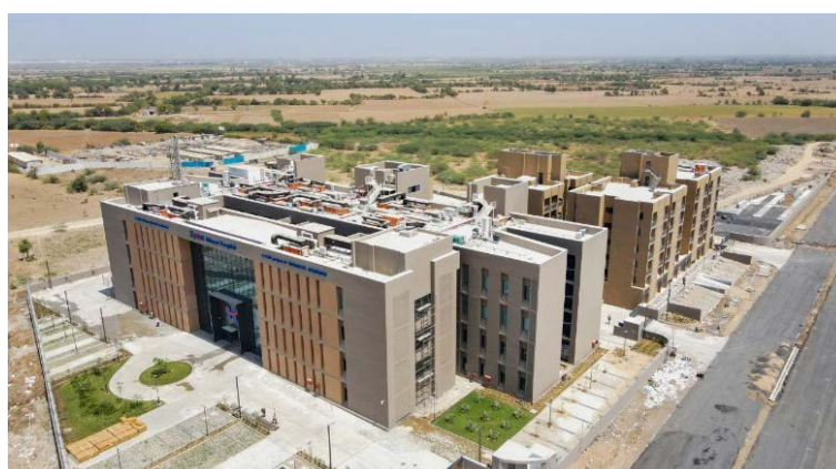
Construction of a general hospital in Gujarat, India
