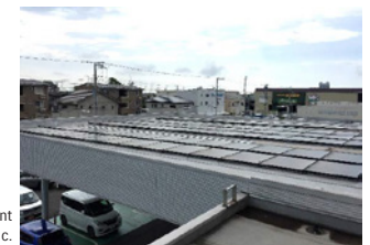
Installing solar power generation equipment Suzuki Motor Sales Keiyo Inc.
