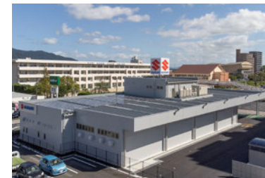
Installing solar power generation equipment Suzuki Motor Sales Shimane Inc.
