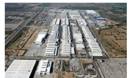
33 SUZUKI MOTOR GUJARAT PRIVATE LIMITED (Gujarat Plant)
